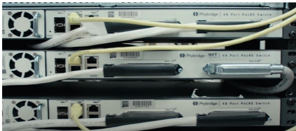
The PoLRE Switches Installed in a Standard 19" Rack
