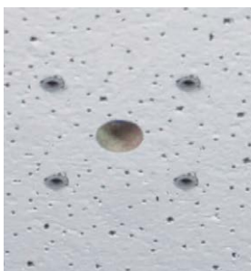
Fig. 14: Holes ready for mounting
