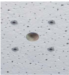
Fig. 16: Holes ready for mounting
